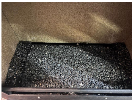
Fig.11 Add vermiculite to mesh trims
