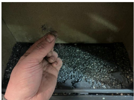
Fig.12 Add slate chips
